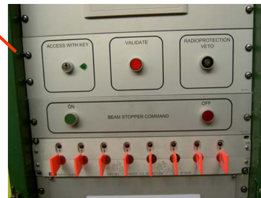
Various controls and key distributor
