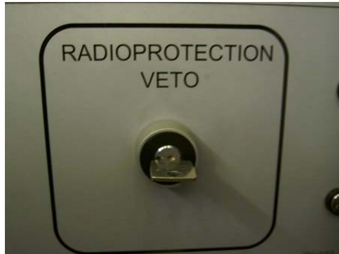
Radio Protection Veto command
